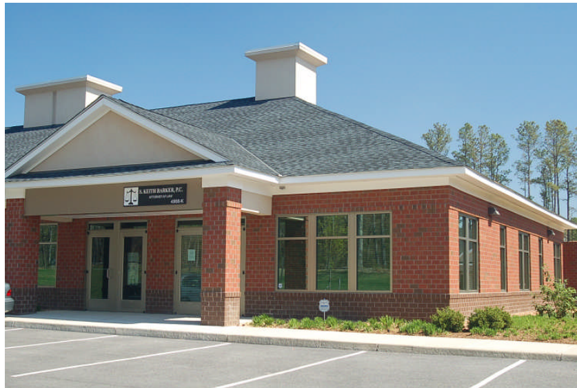
Our office - 4908 Dominion Boulevard, Suite K in the Dominion Place section of The Innsbrook Office Park
